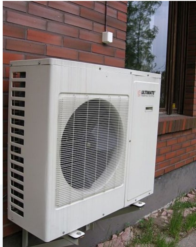
New geothermal heat pump
