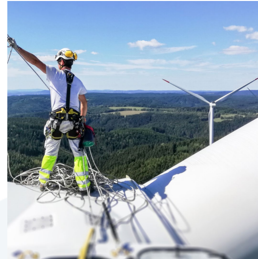
Wind turbine maintenance
